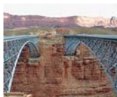
Hoover Dam Bridge
